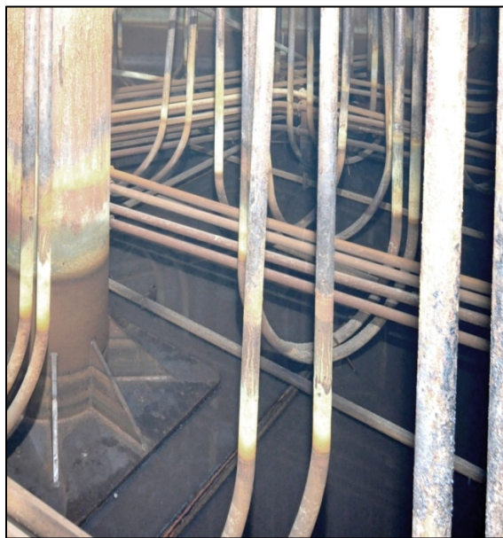
Figure 3.5-2: Photograph of Tank 12H Primary Tank Floor (After Waste Removal in September 2013)
