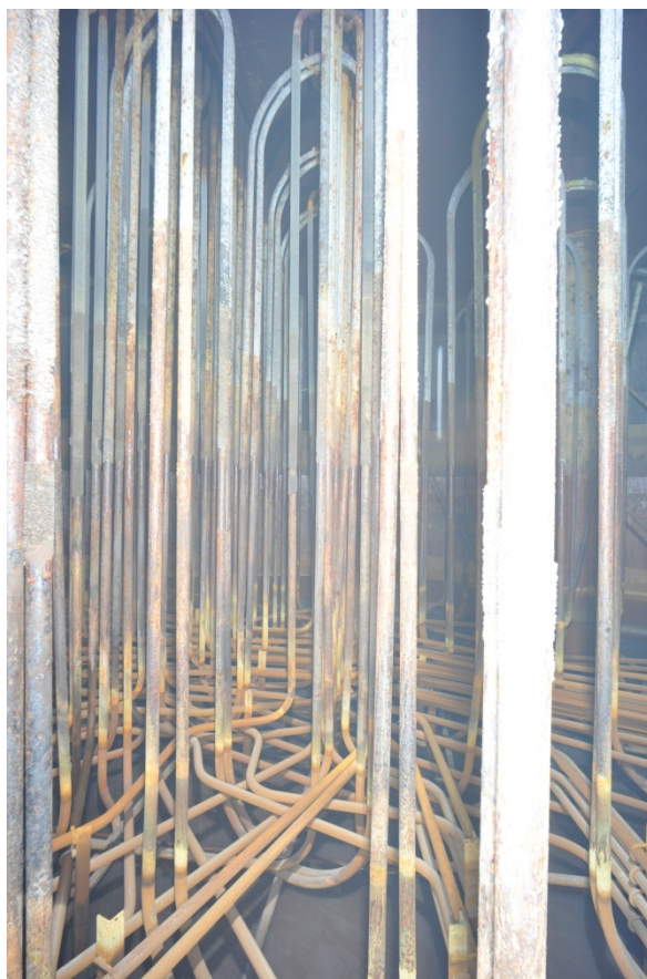
Figure 2.1-3: Tank 12H Cooling Coils
